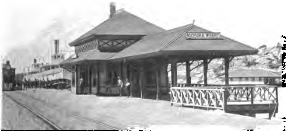
MUSKOKA WHARF STATION.
